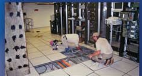
Computer Room Decontamination & Super Cleaning
